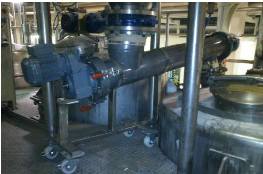
Easy clean screw conveyor AB Food (Thailand) Ltd. / Ovaltin Sugar + Malt + Milk powder
